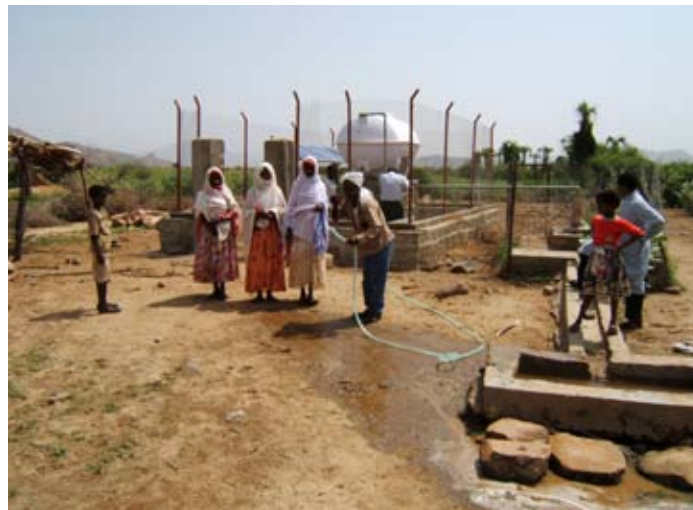
Shekloti water project (2005)
