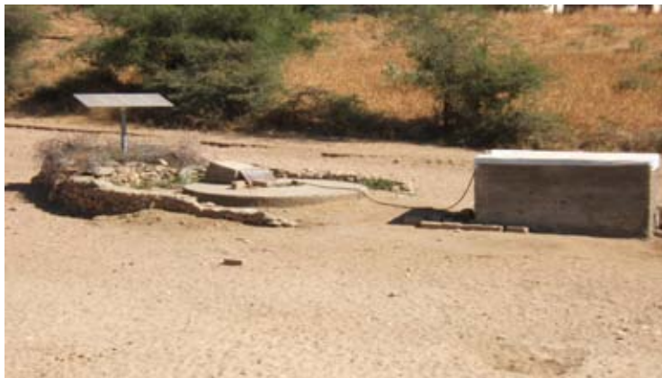
Shnara well powered by solar cells (2004)
