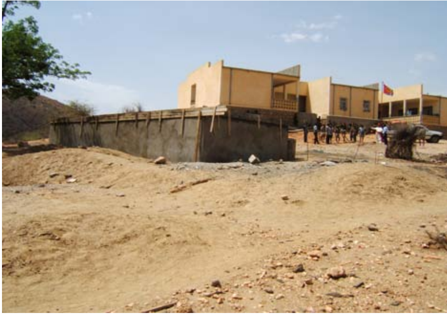
Ygear water reservoir for school Completed on September 2005
