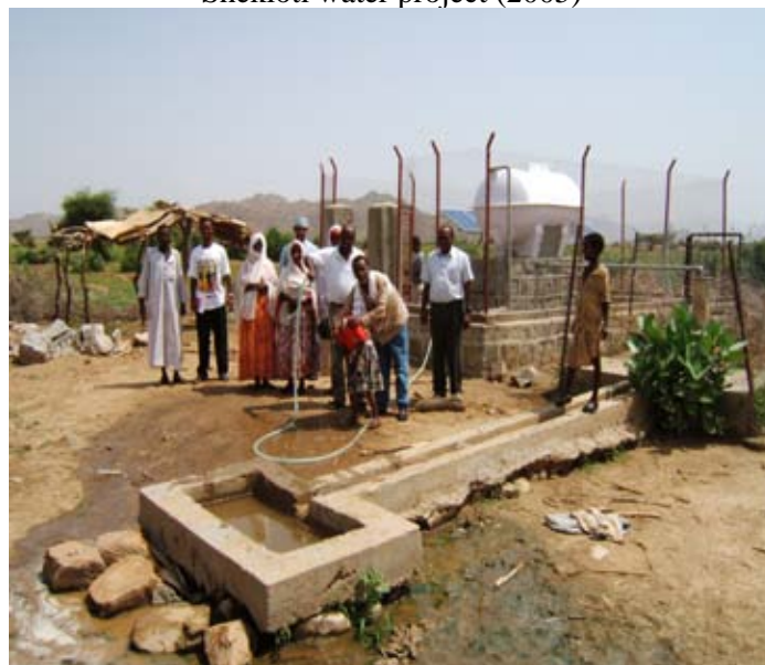
Shekloti water project (2005)
