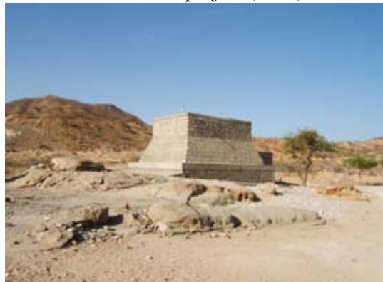
Jufa Water reservoir (2005)
