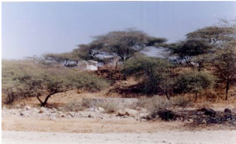
Well and power generation center for Brekentia (2001)
